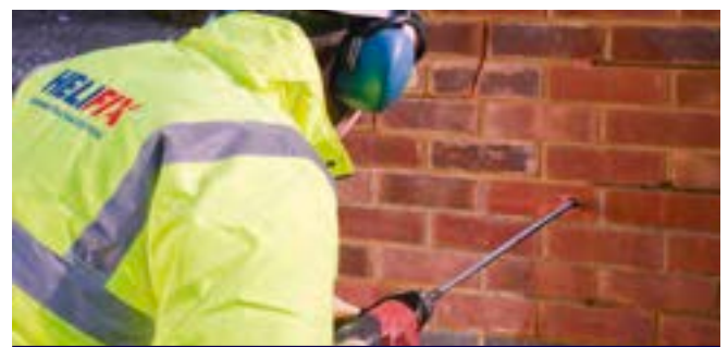
Drilling clearance hole for installing BowTie into joist end
