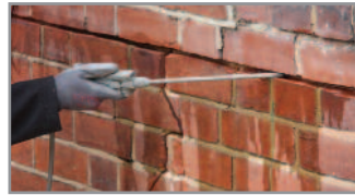
2. Clean out slots and flush with clean water and thoroughly soak the substrate within the slot
