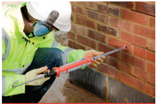
Injecting resin to complete the RetroTie installation
